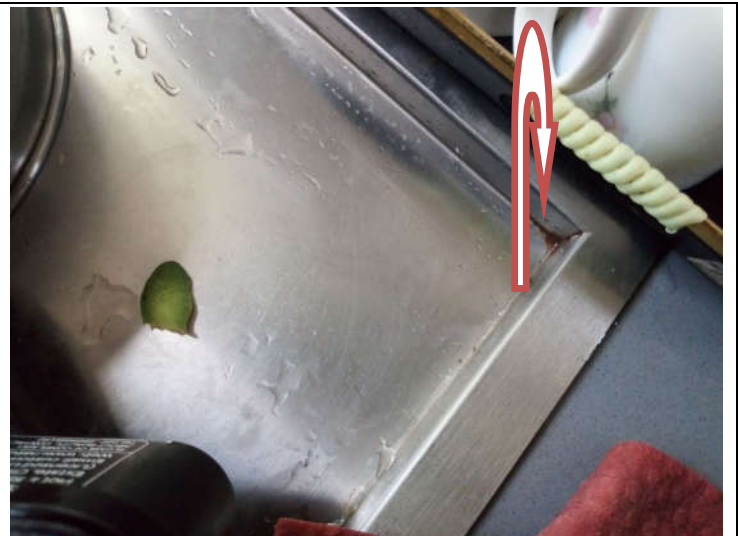
Oxidized in the corner because user leaves the corner too wet with water on the surface for a long time without cleaning it. Iron deposits can occur.
